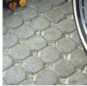
In order to reduce stormwater runoff from your lot, minimize the amount of paving or consider a pervious paving system that would allow rainwater to infiltrate into the ground.
